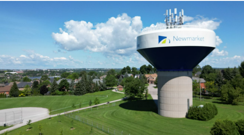
Ivsbridge Elevated Tank, Town of Newmarket
