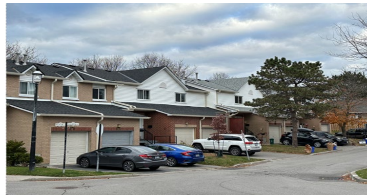
Roof downspout and eavestrough replacement Mulock Village, Town of Newmarket
