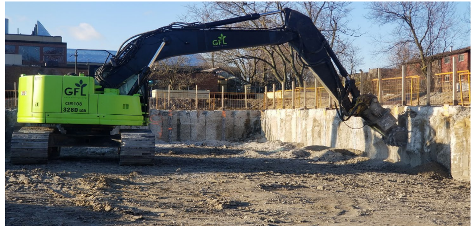
Excavation for foundations
