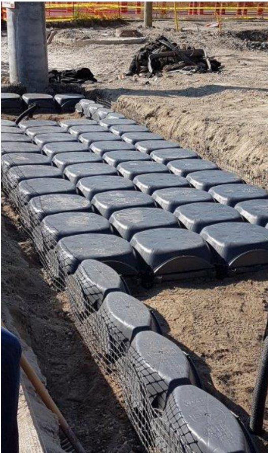
Installation of a soil cell system
