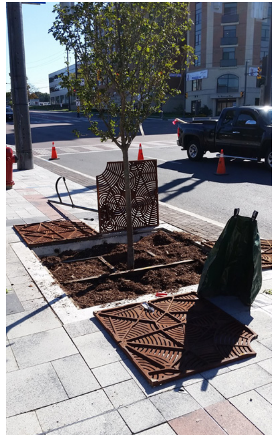
Tree grate installation
