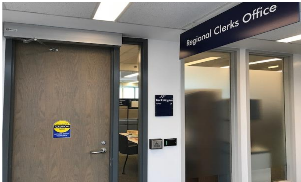
Figure 1 Installation of Power Door Operator
