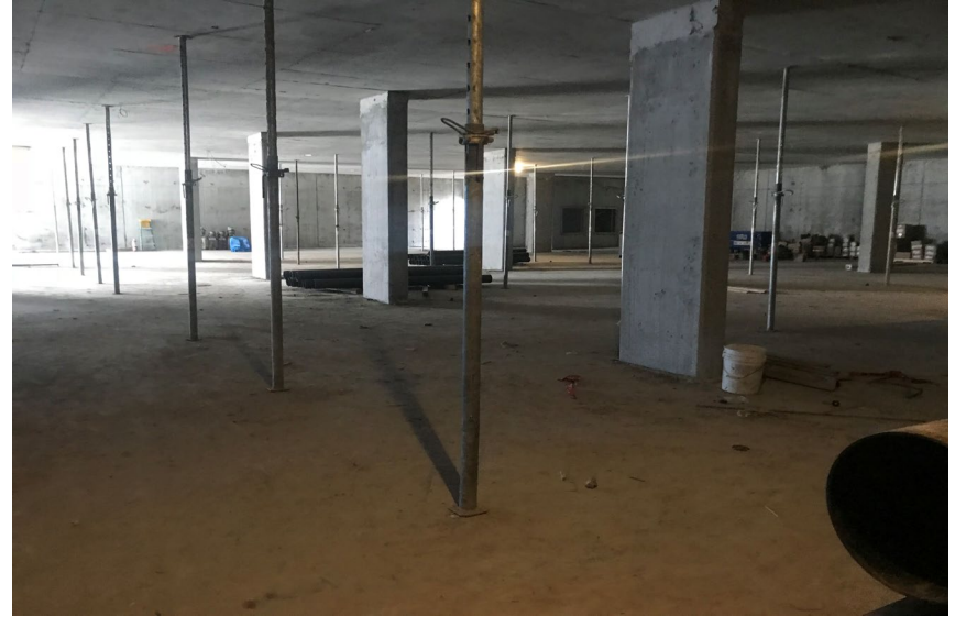
P1 underground parking
