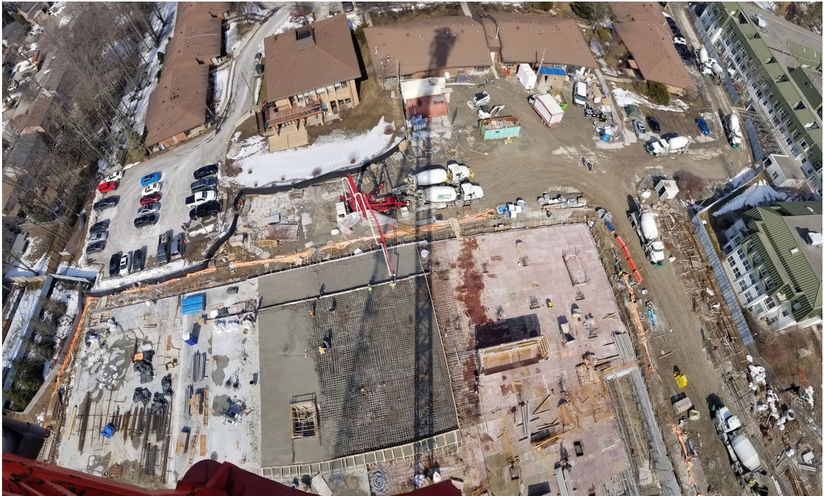
Ground floor slab and garage roof
