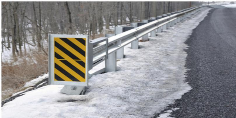
A recent example of the implementation of guardrail barriers with end treatments is the installation on the north side of Lakeshore Road, completed as part of the shoreline stabilization project. Staff will continue to consider clear zones and guardrail barriers as part of future road reconstruction, shoreline stabilization, new development, and other opportunities as appropriate.
