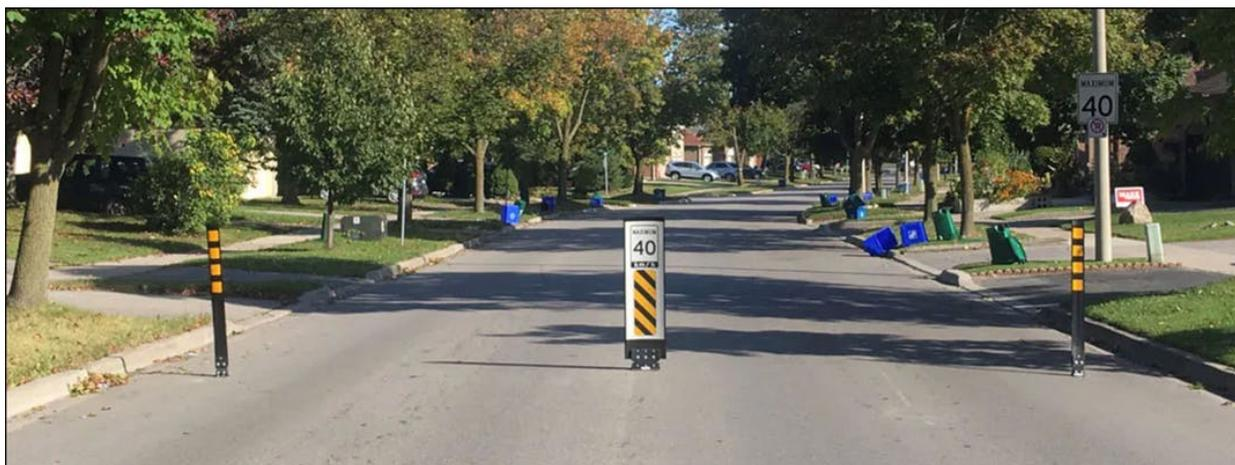
The Town implemented a traffic delineator pilot project in 2019, consisting of the installation of delineators in four school zone locations. Staff monitoring of the traffic delineators indicated lower vehicular speeds in their vicinity. Resident feedback obtained through a survey indicated 85% of respondents felt the delineators had a positive effect on reducing traffic speed, and 74% of respondents were in favour of their continued use.
