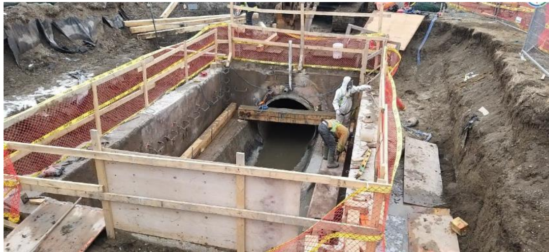
Leslie Gravity Sewer and Chamber Rehabilitation
