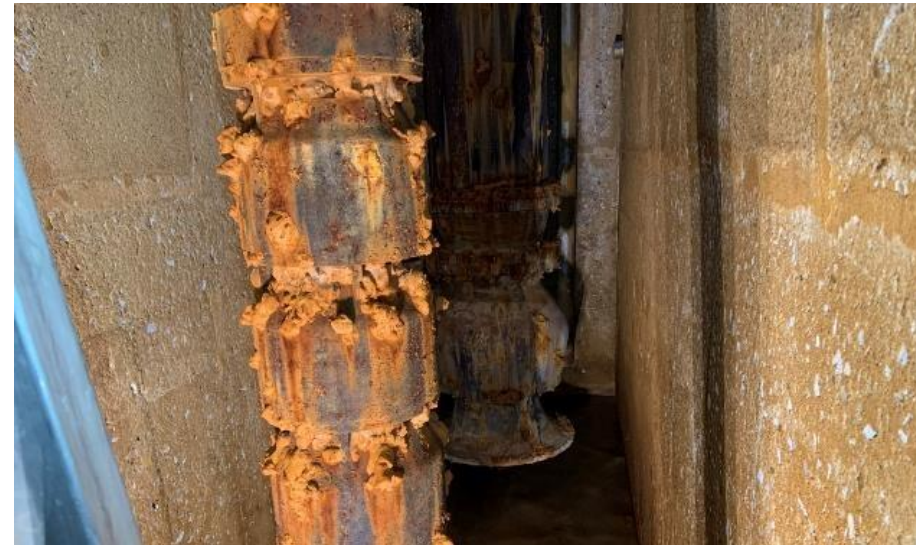
Tubercule corrosion on pump columns
