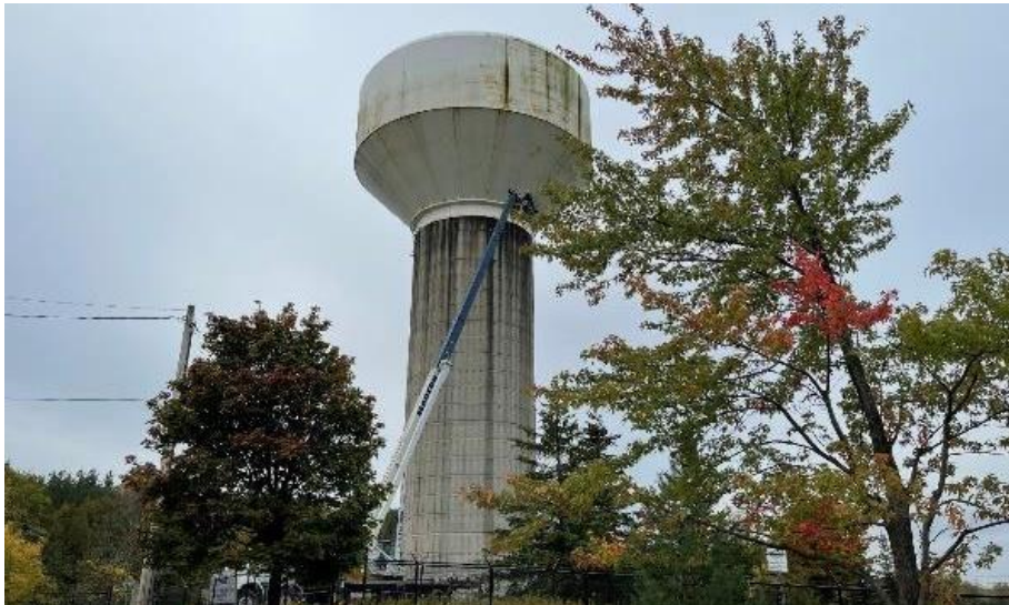
Tank coating delamination and steel corrosion on elevated tank
