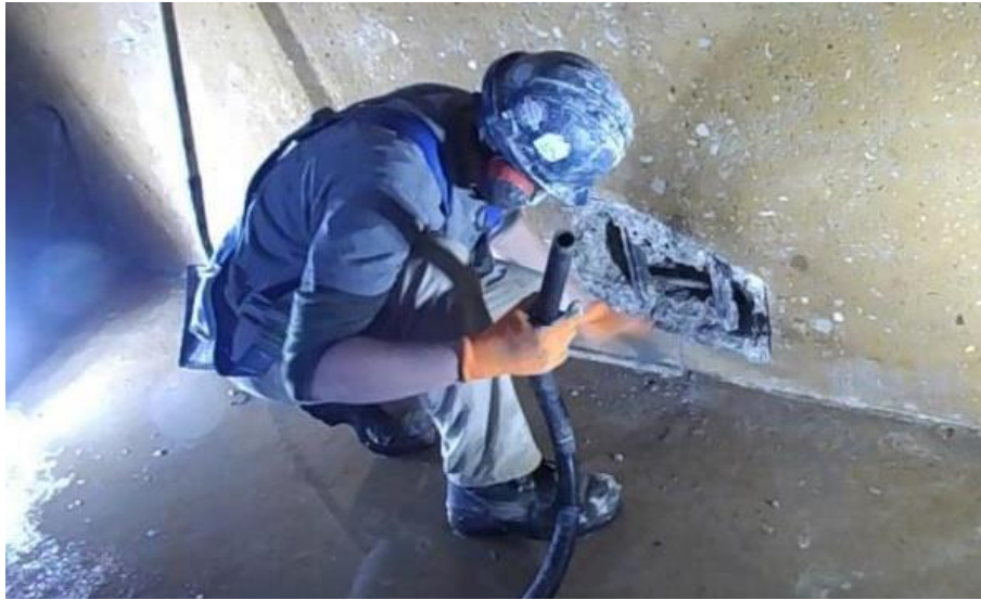
Concrete repairs inside reservoir
