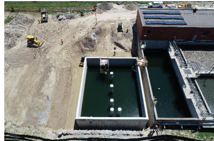
Sutton WRRF Upgrades - Equalization Tank
