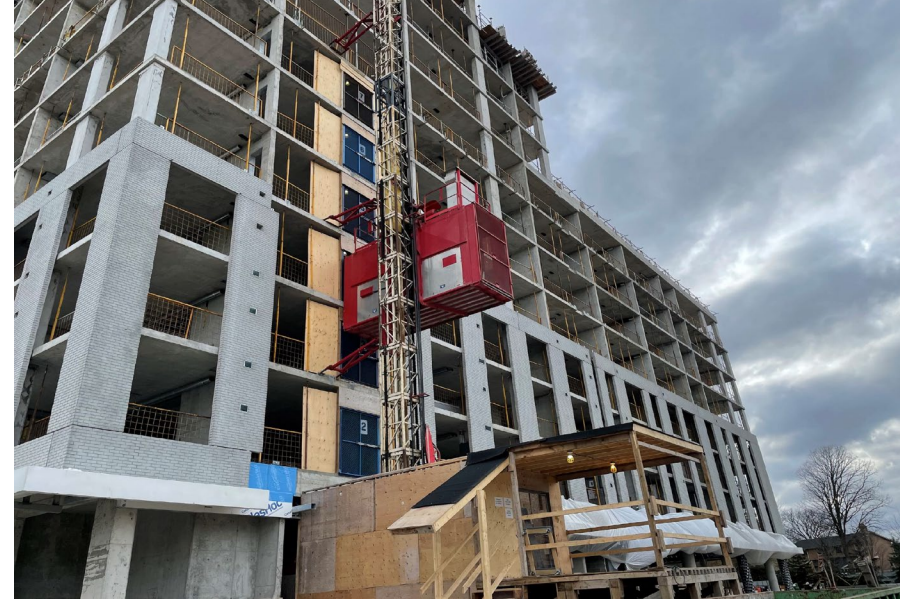
View showing hoist along north elevation
