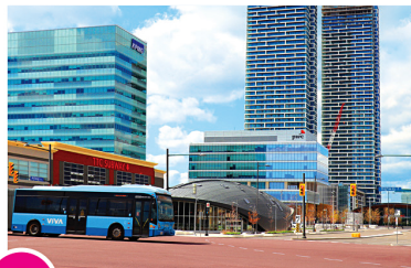
2 Vaughan Metropolitan Centre
