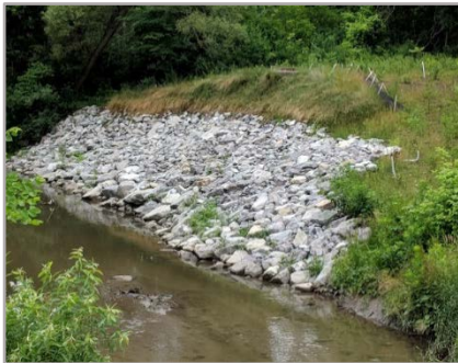
(German Mills, Emergency Bank Stabilization)
