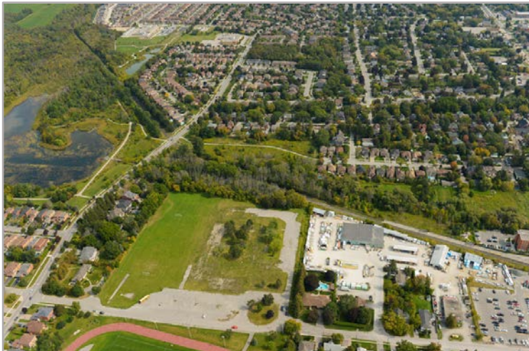
(Stouffville Dam, Aerial photo)
