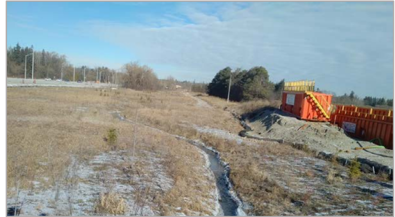
(Bayview Avenue, Pre-Construction)
