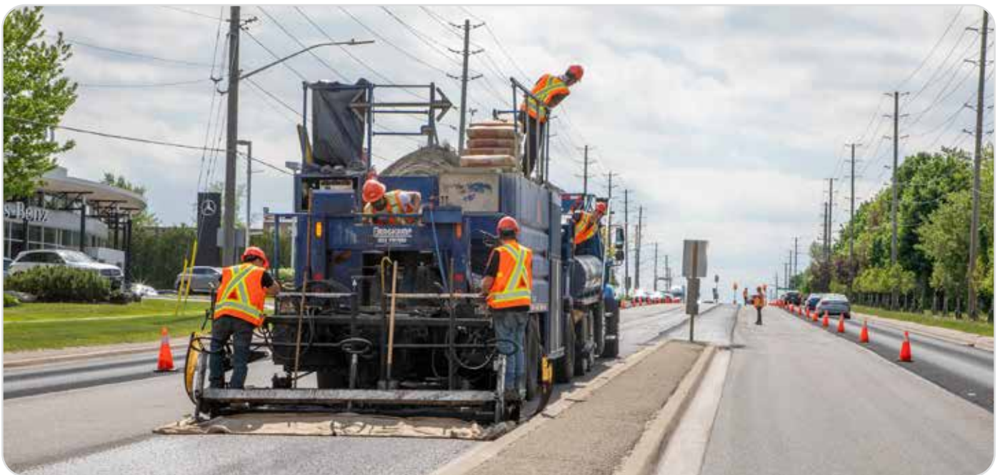
▲ Resurfacing of Mulock Drive, East of Yonge Street in the Town of Newmarket.
