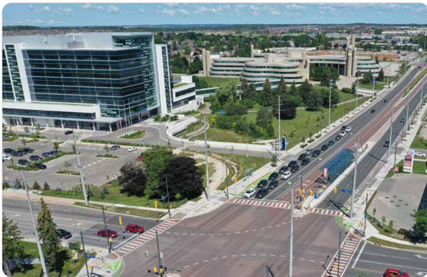
▲ Aerial view of Yonge Street and Eagle Street intersection in the Town of Newmarket.
