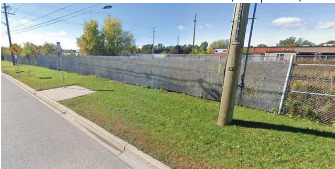
Reinforced Chain Link Fence down Cousins Drive as of June 3, 2020
