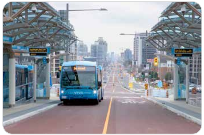
▲ Bus serving travellers at Vivastation along Yonge Street in the City of Richmond Hill.
