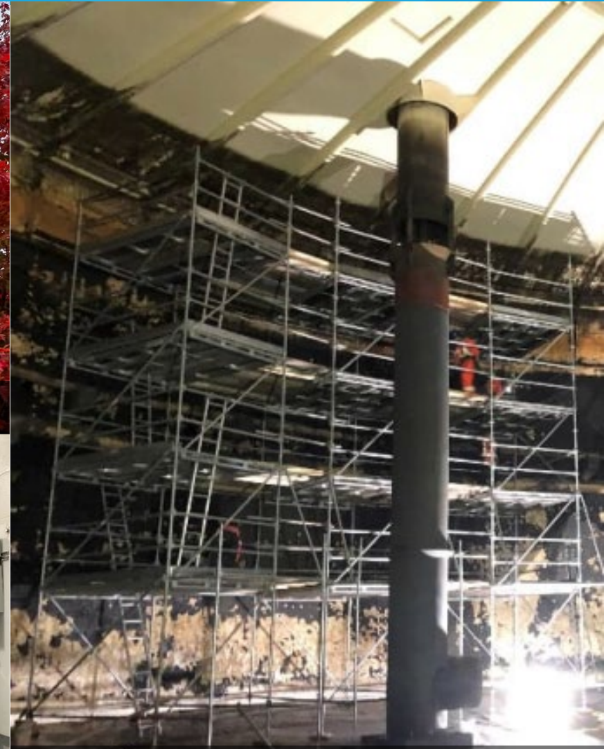
Scaffolding at Primary Digester and Coating Inspection, Duffin Creek, City of Pickering
