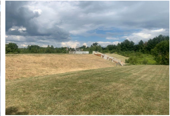
Stouffville Dam Post Embankment Maintenance
