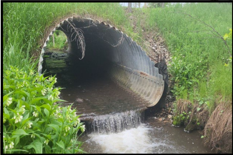
Before culvert replacement
