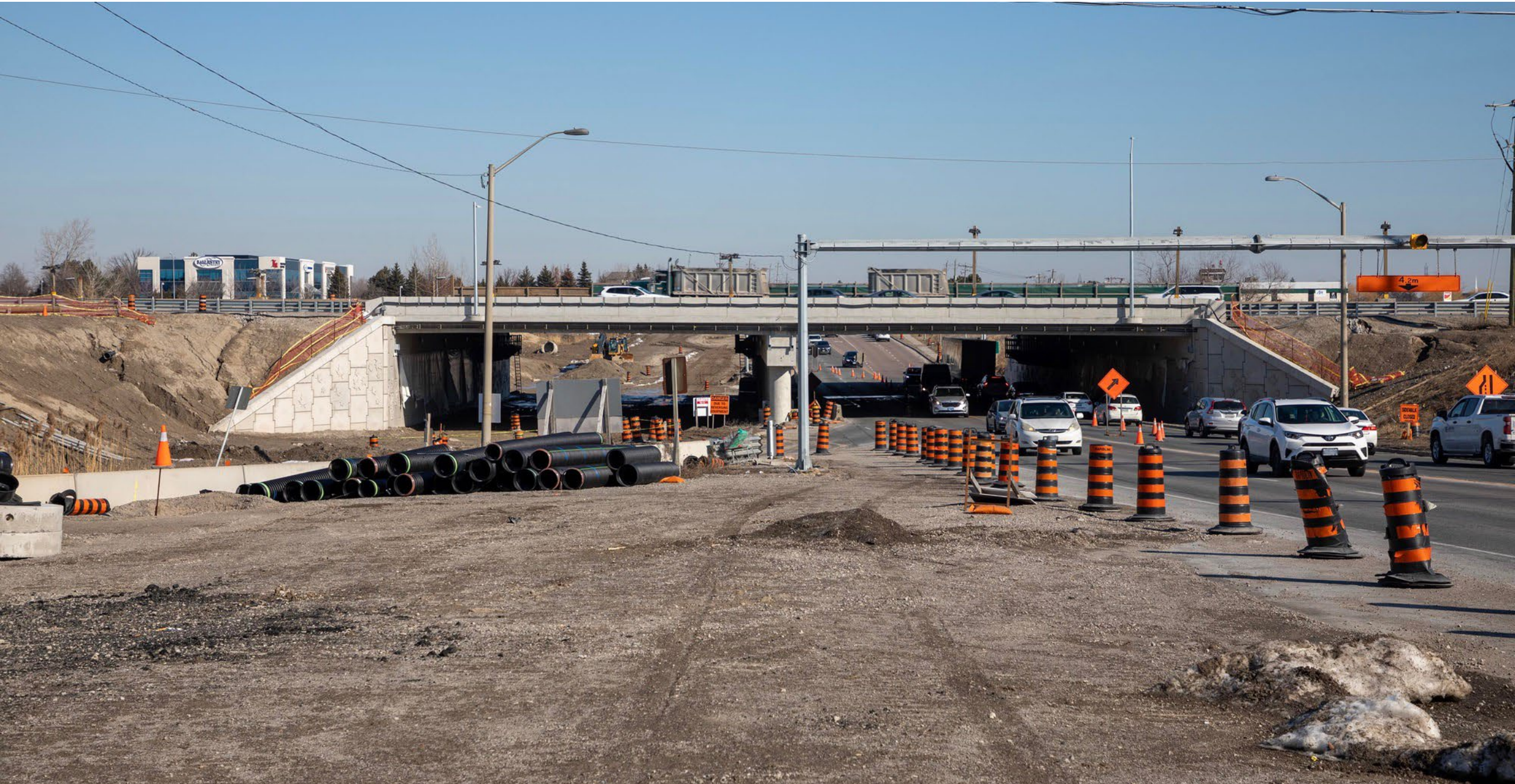
Construction of new, widened Highway 404 bridges over 16th Avenue
