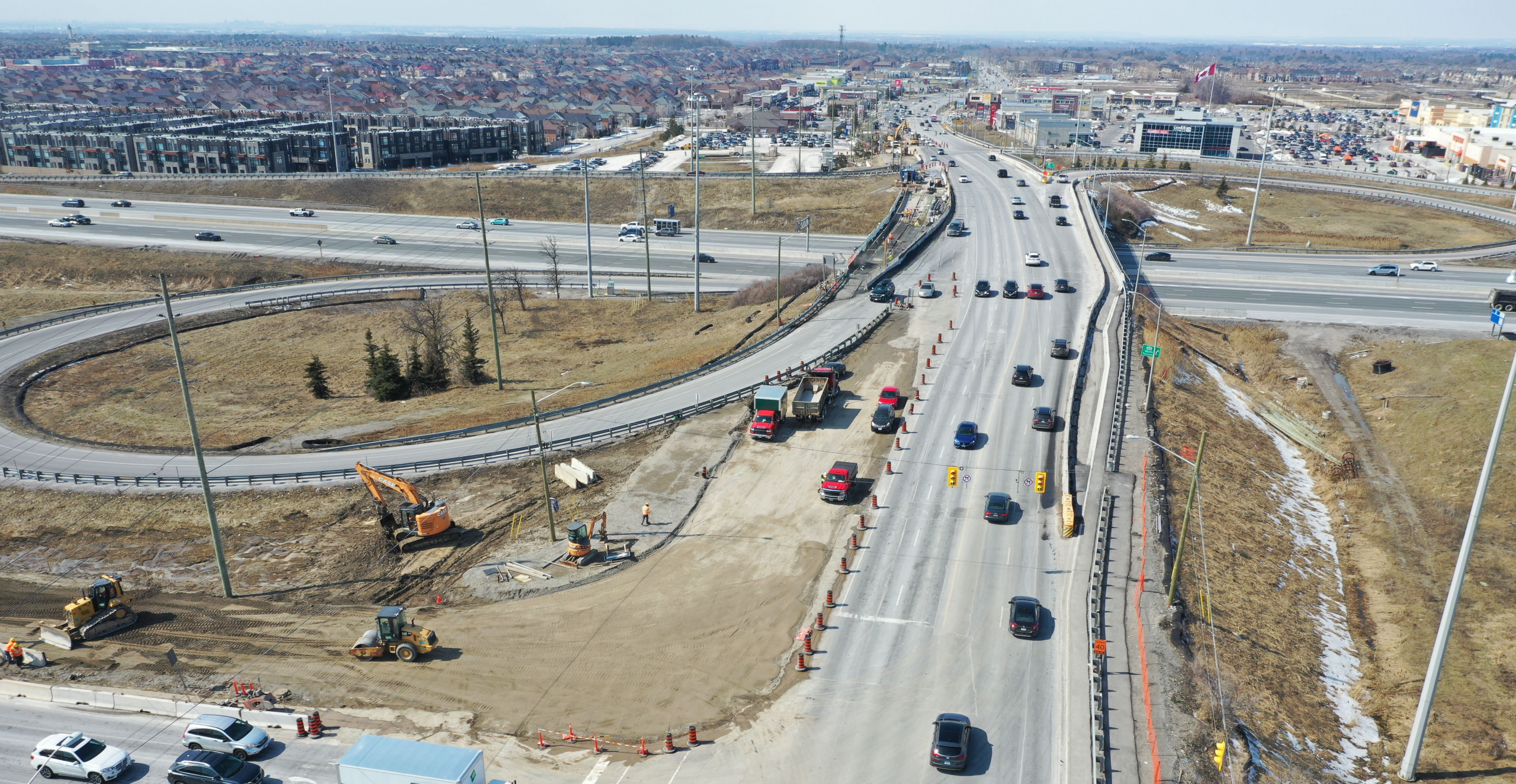
Widening of Major Mackenzie Drive over Highway 400 interchange under construction
