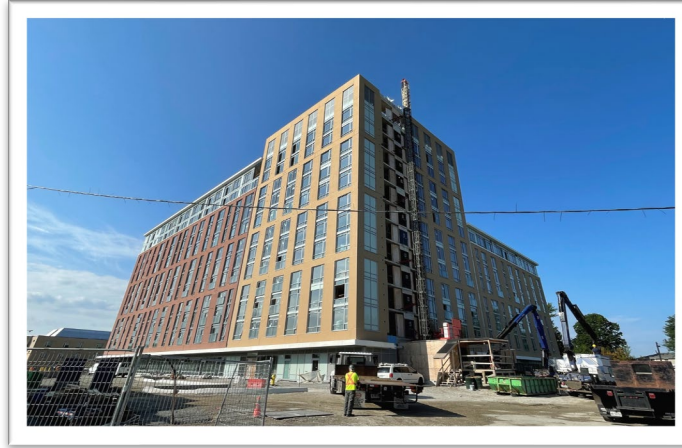
Unionville Commons, 265 units City of Markham
