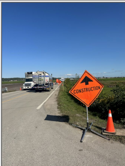
Jane Street at South Canal Bank Road, King
