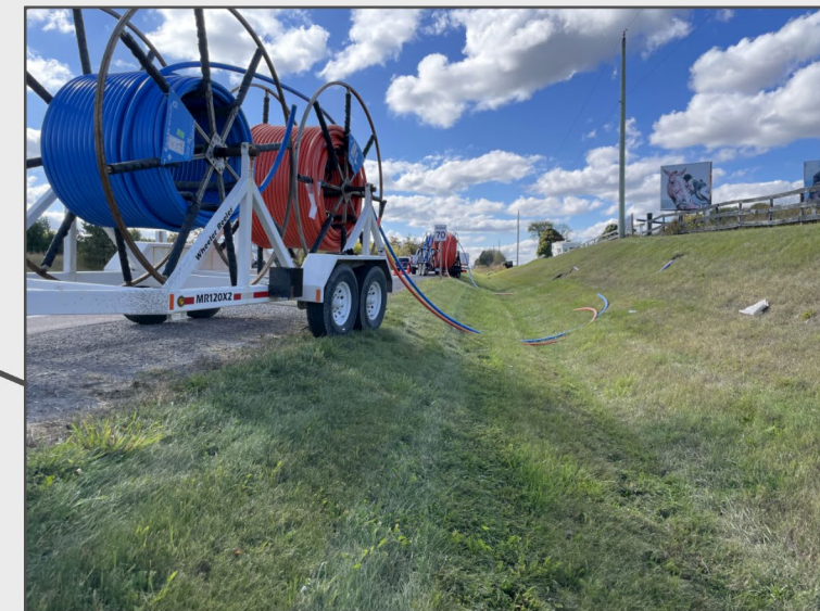
Davis Drive between Kennedy Road and McCowan Road, East Gwillimbury
