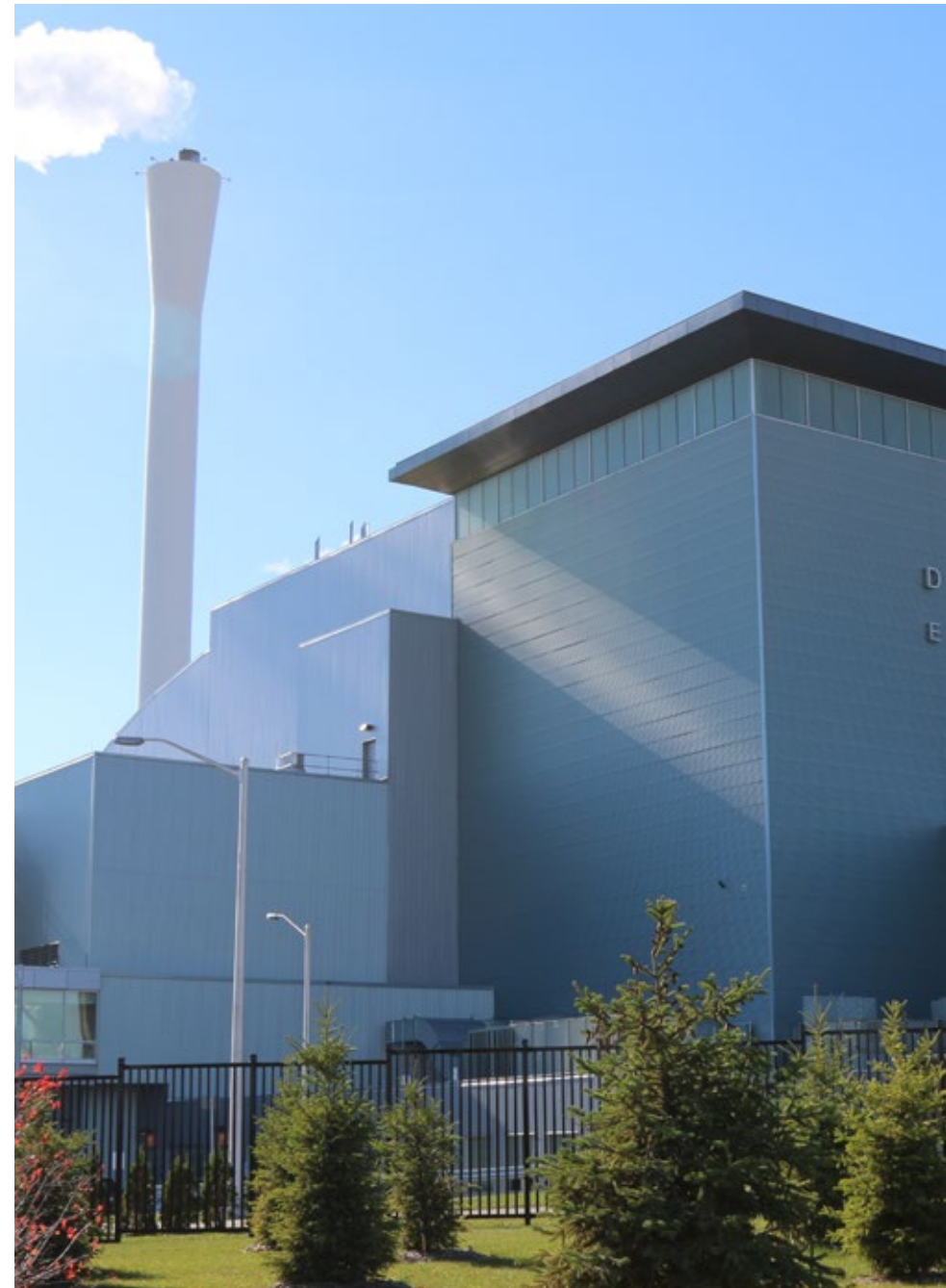
Durham-York Energy Centre
