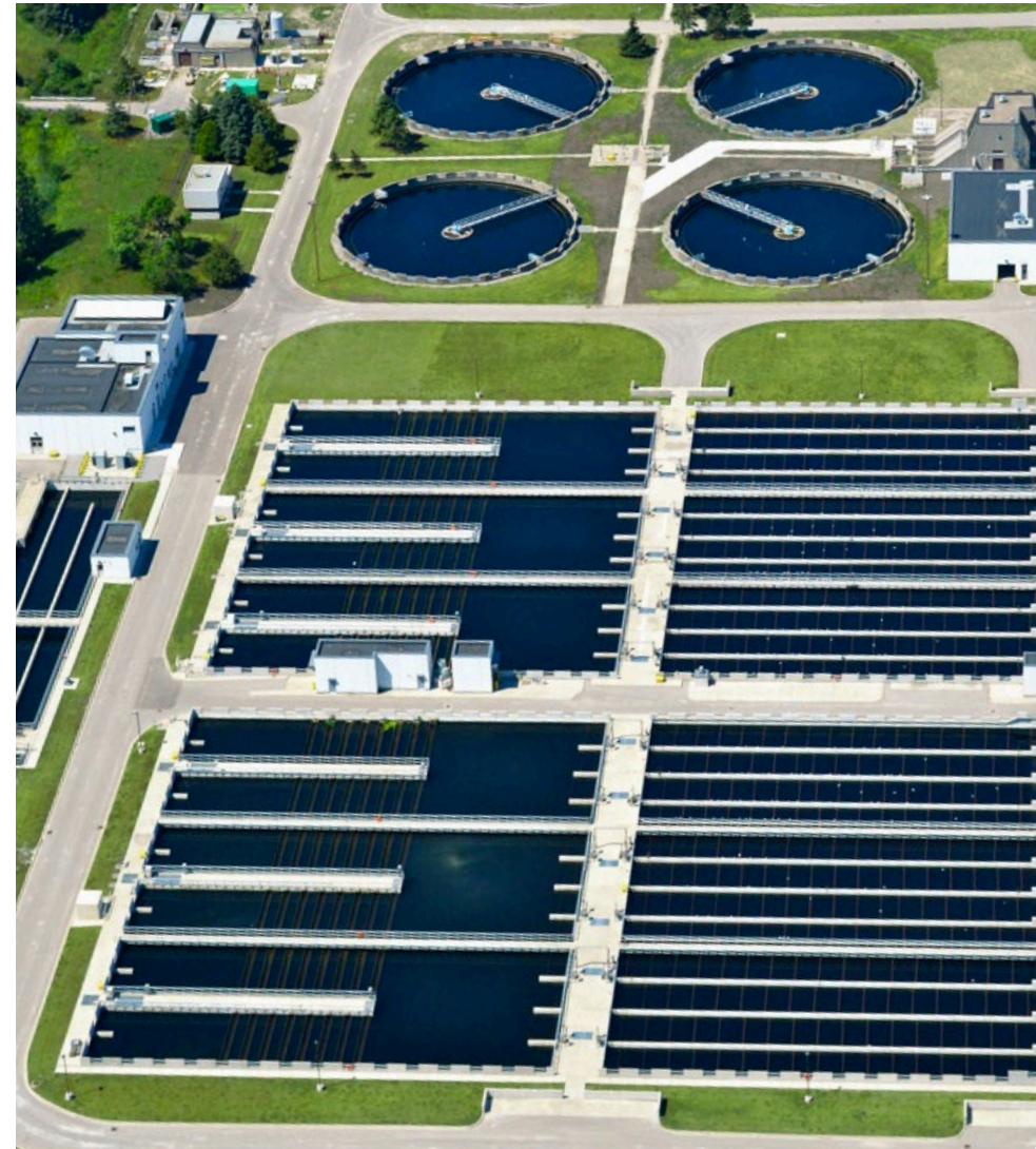
Duffin Creek Water Pollution Control Plant
