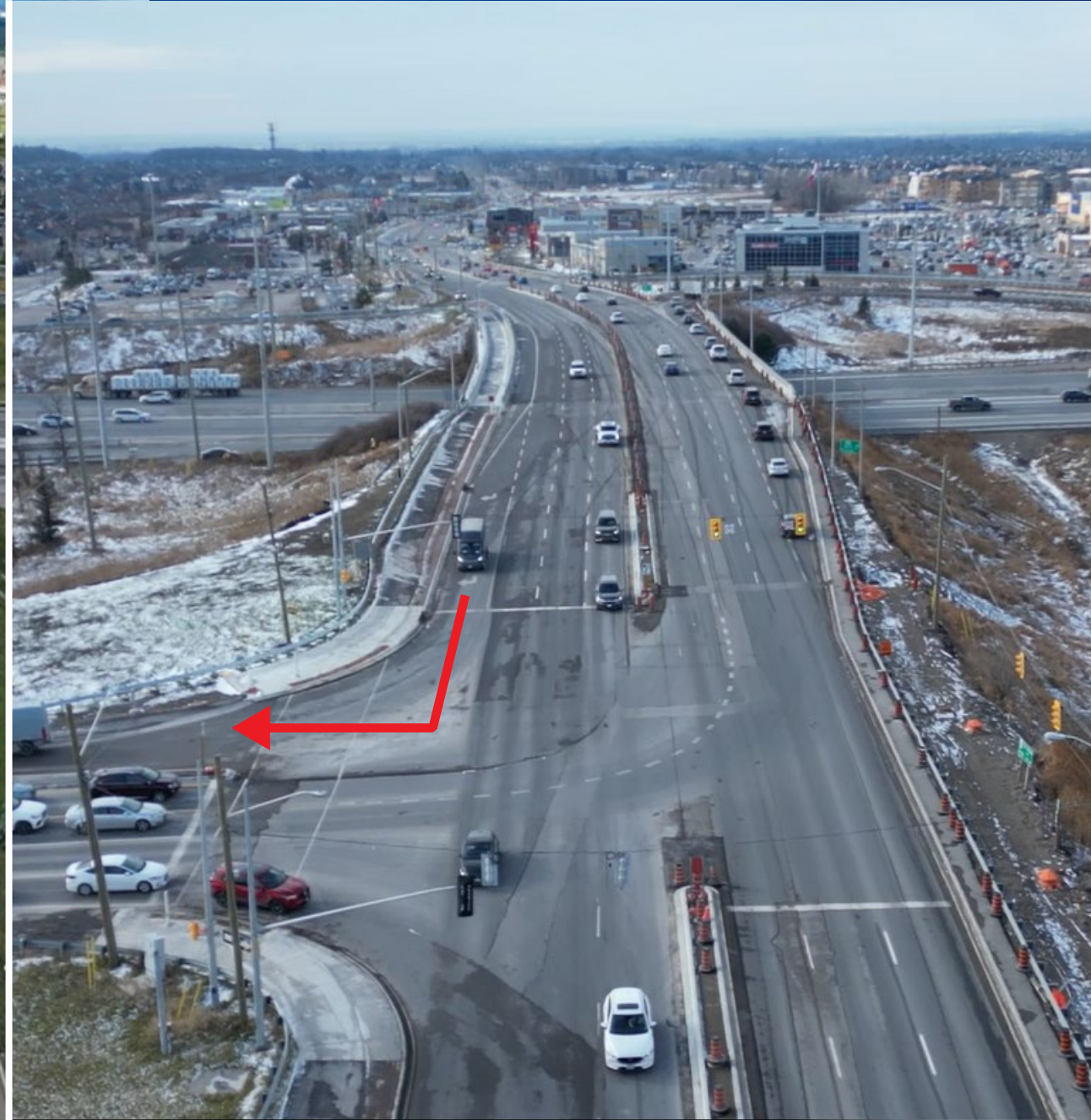
After: Highway 400 on-ramp relocated to signalized intersection
