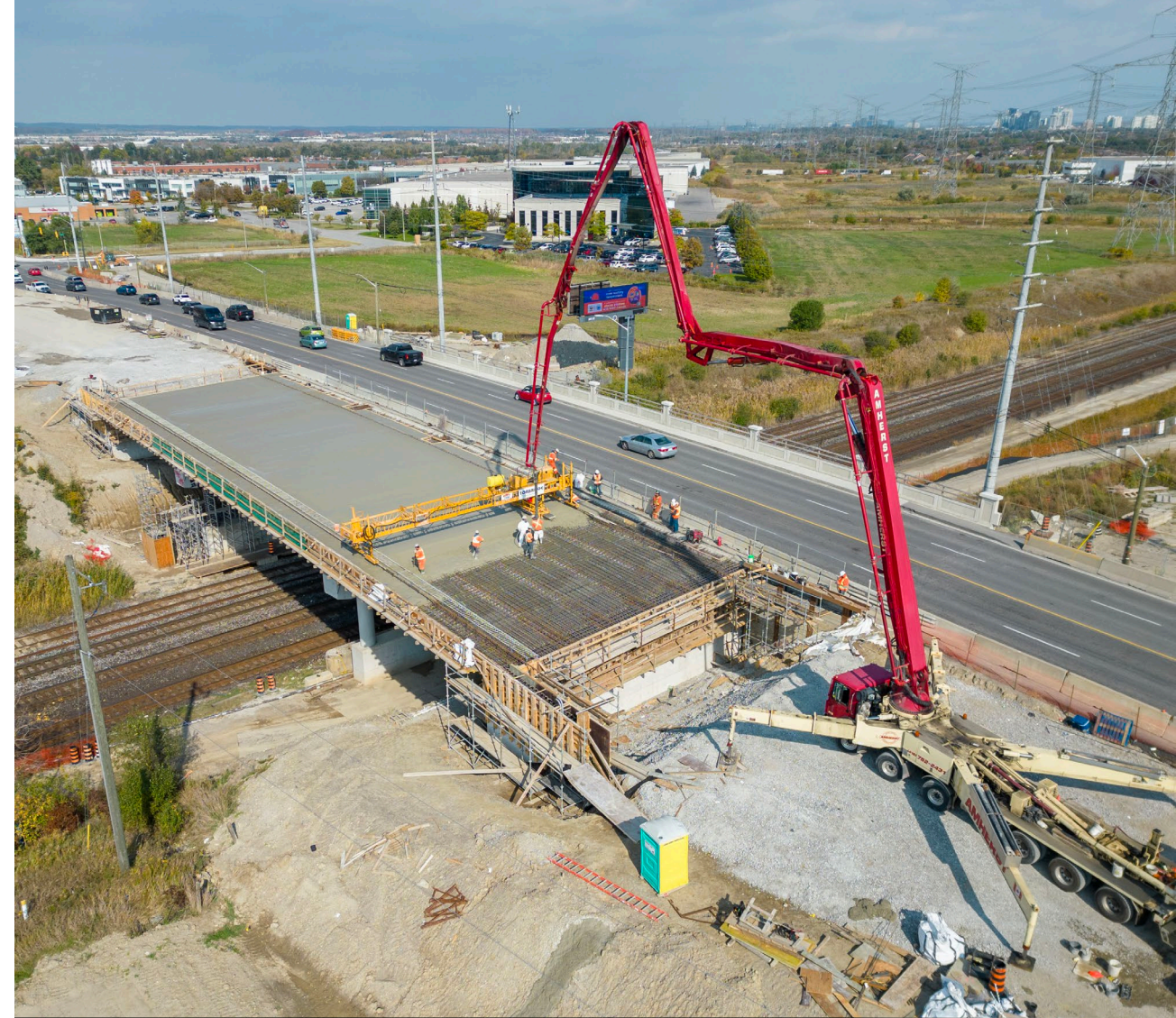
Keele Street, south of Highway 407, City of Vaughan
