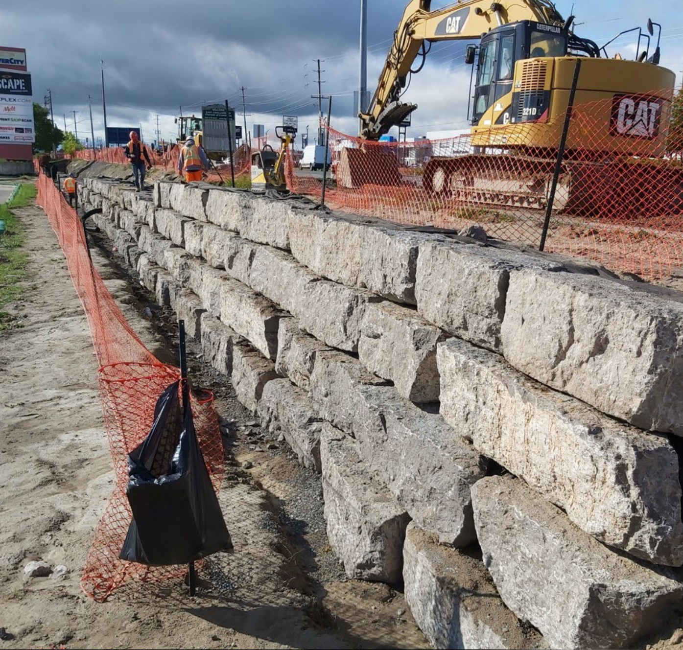
New retaining wall along Yonge Street, Town of East Gwillimbury
