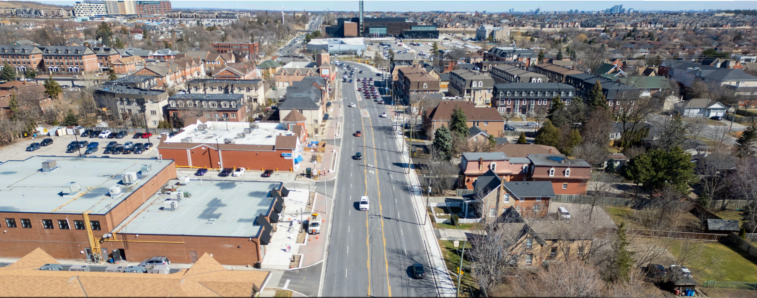
New centre-turn lane on Major Mackenzie Drive, looking east toward Keele Street, City of Vaughan
