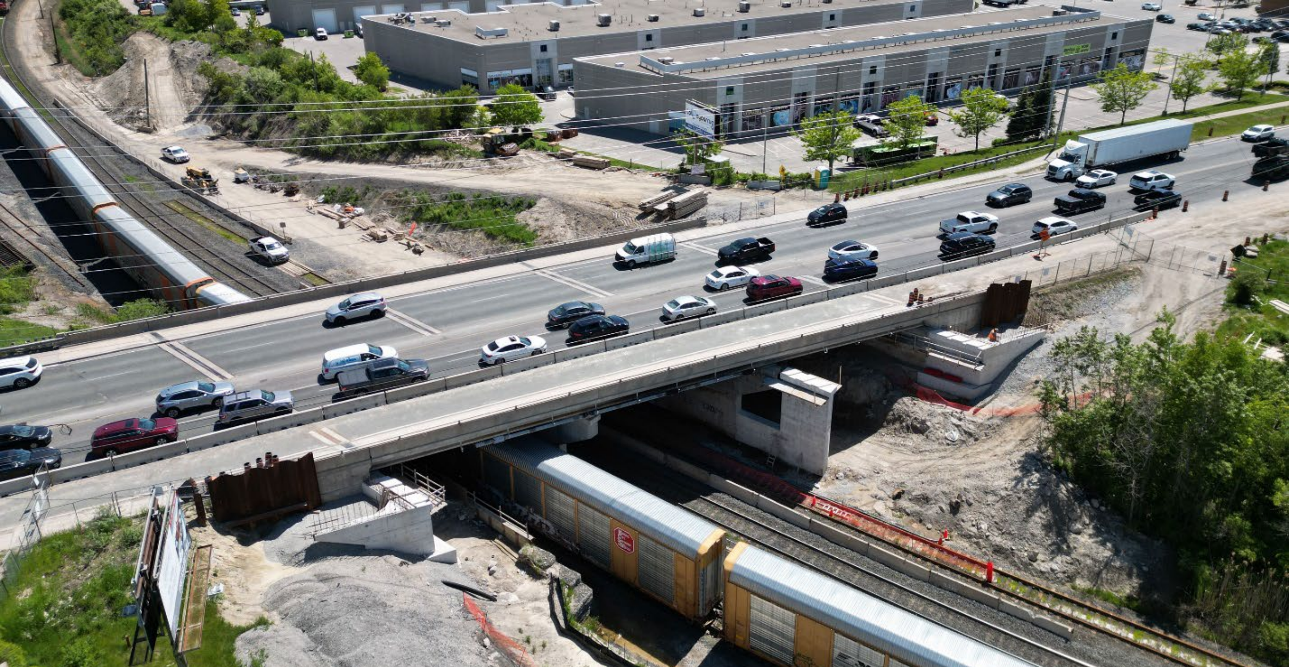
Aerial view of work to widen the CN Rail bridge on Rutherford Road, east of Melville Avenue/ Creditstone Road, City of Vaughan
