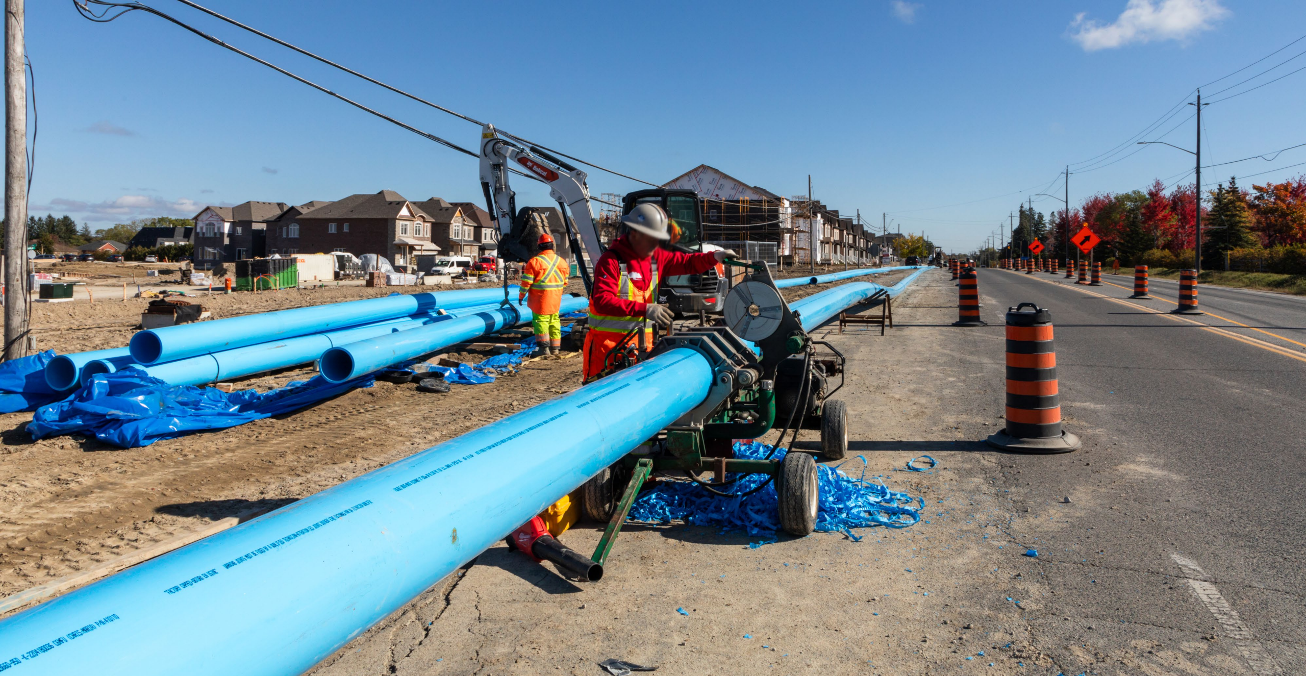
Watermain installation on King Road, City of Richmond Hill
