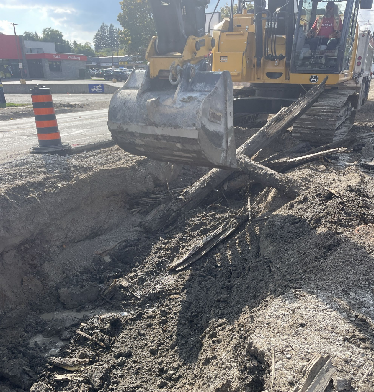
Discovery of wooden corduroy road constructed in 1918 below existing asphalt on King Road, City of Richmond Hill
