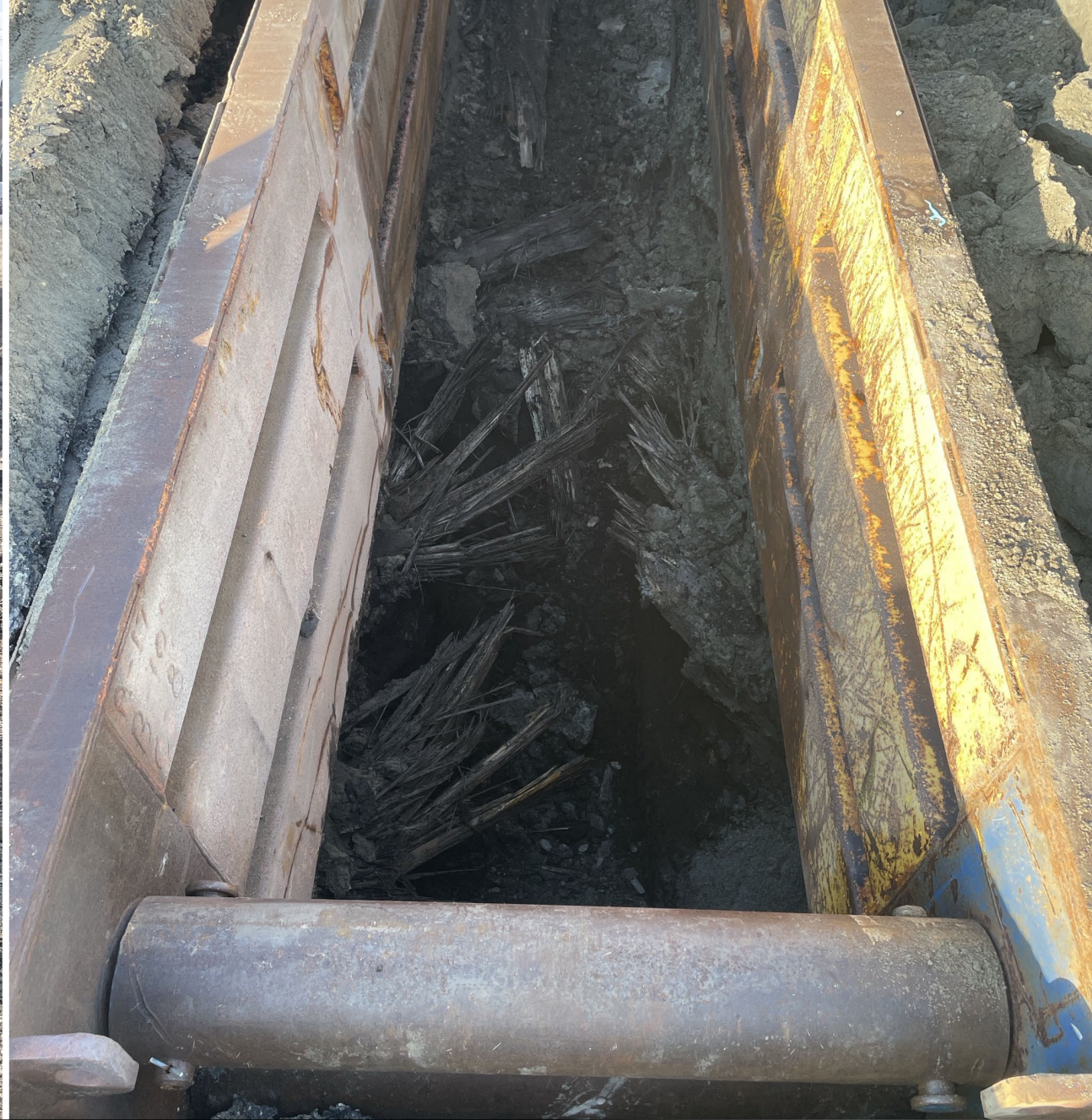
Discovery of wooden corduroy road constructed in 1918 below existing asphalt on King Road, City of Richmond Hill
