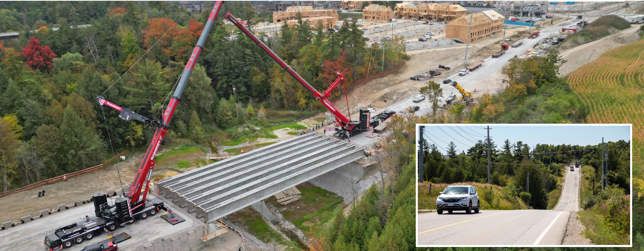
Installation of bridge girders on Teston Road, east of Pine Valley Drive, City of Vaughan
