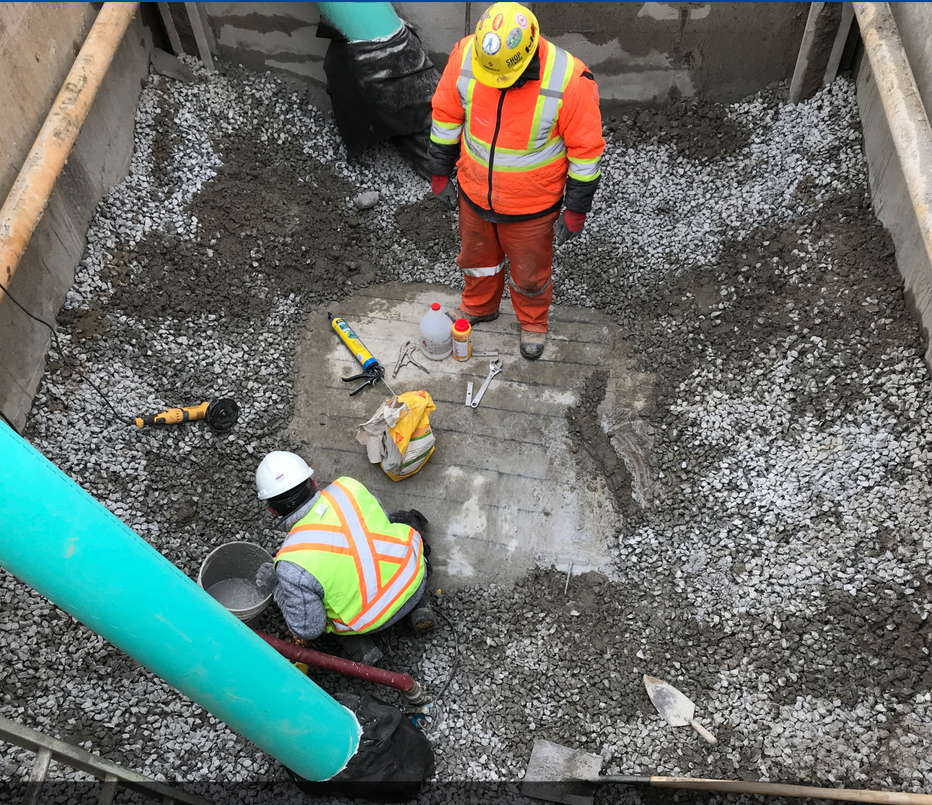
Structural condition assessment on the Primary Trunk Sewer
