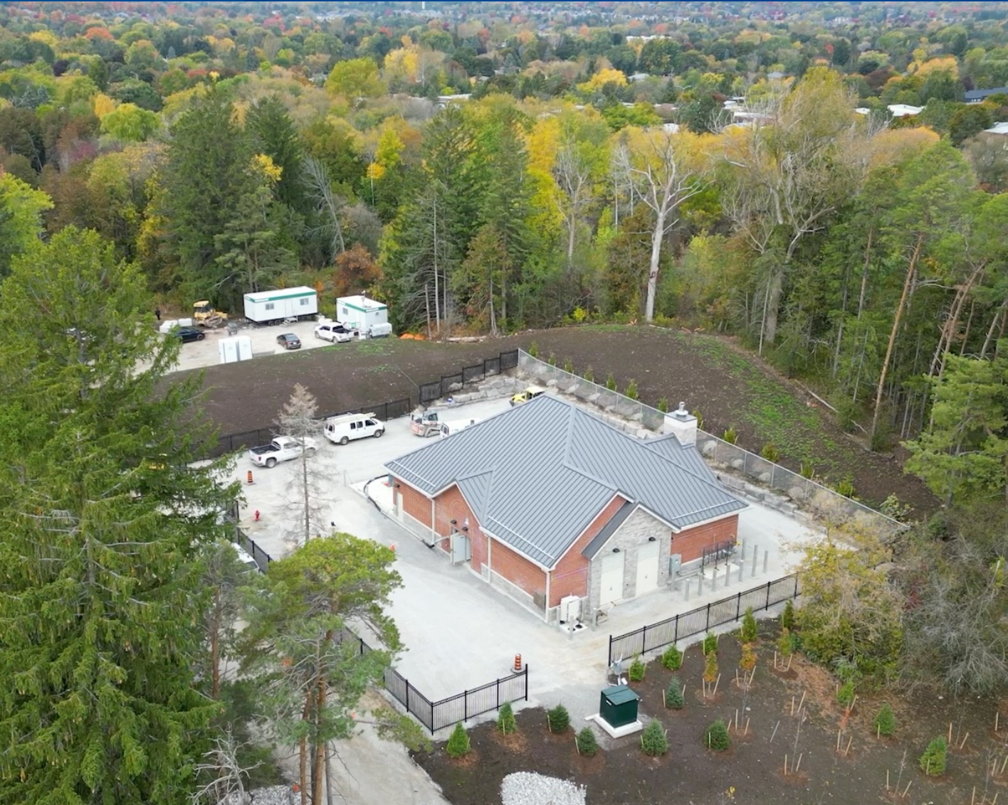
Henderson Pumping Station, Town of Aurora
