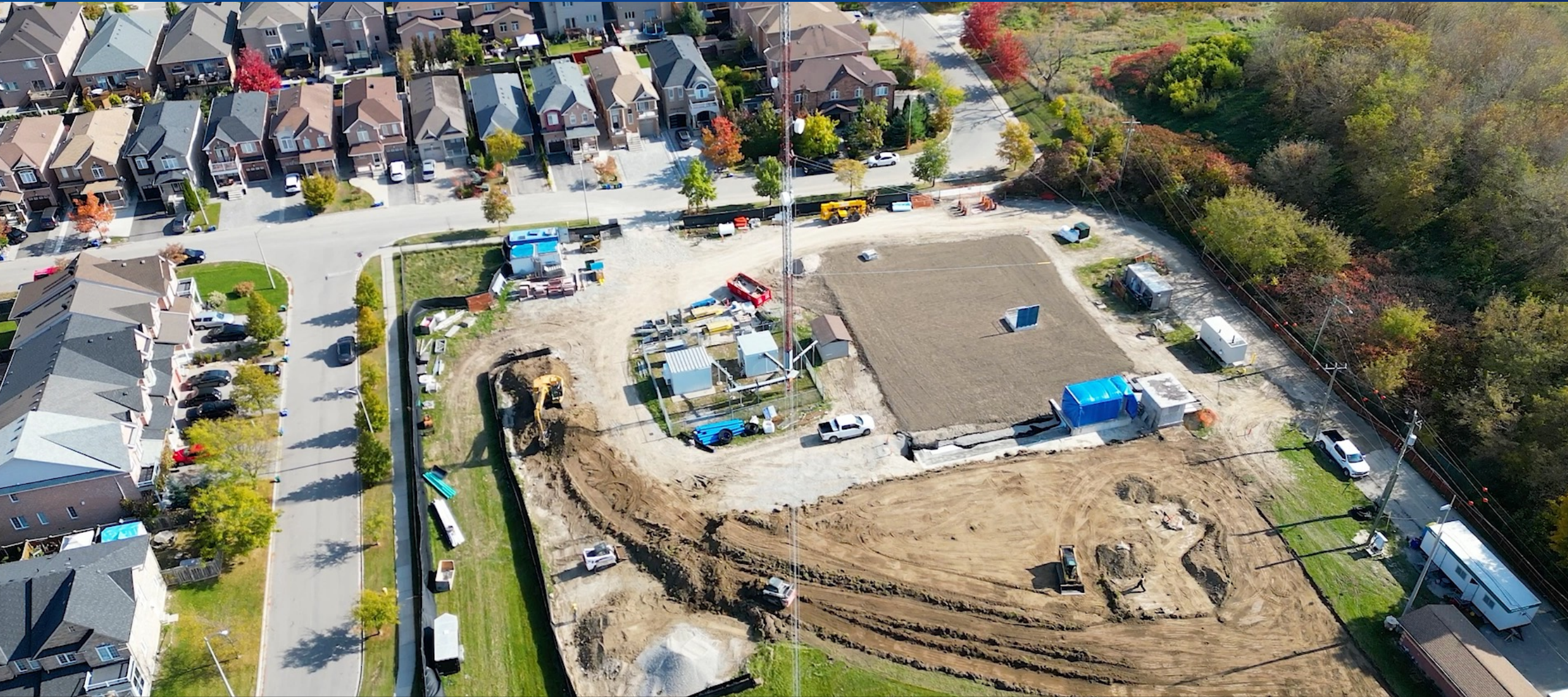
Construction of the Maple North Reservoir, City of Vaughan
