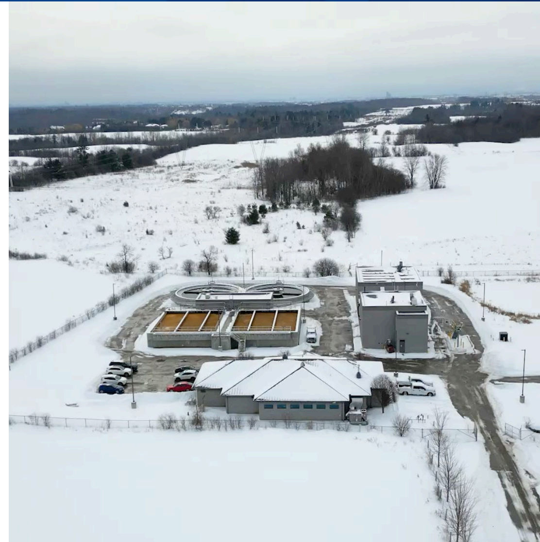
Nobleton Water Resource Recovery Facility, Township of King
