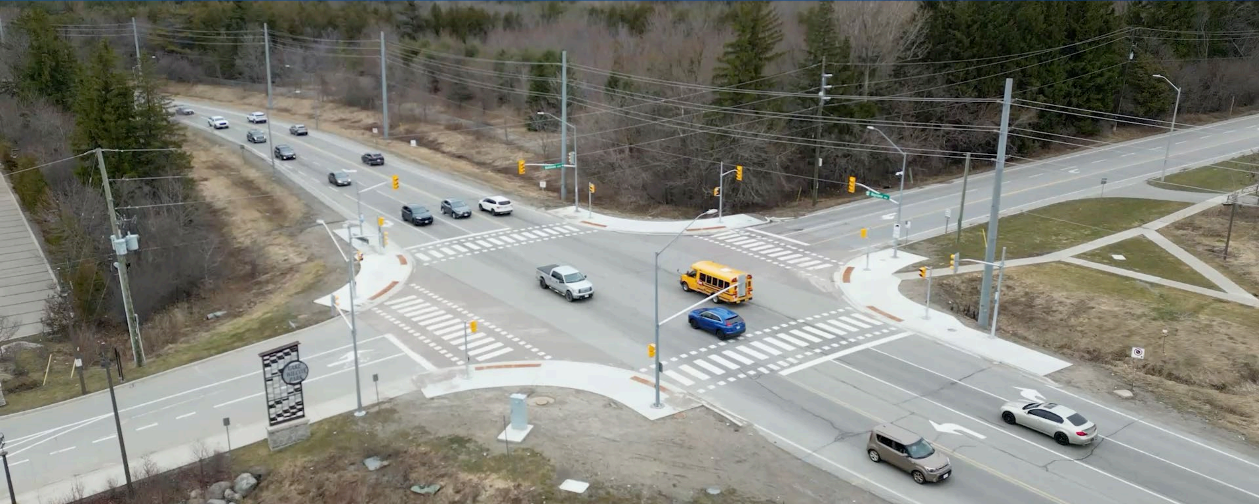
New traffic signal installed at Bayview Avenue and Bethesda Sideroad, City of Richmond Hill
