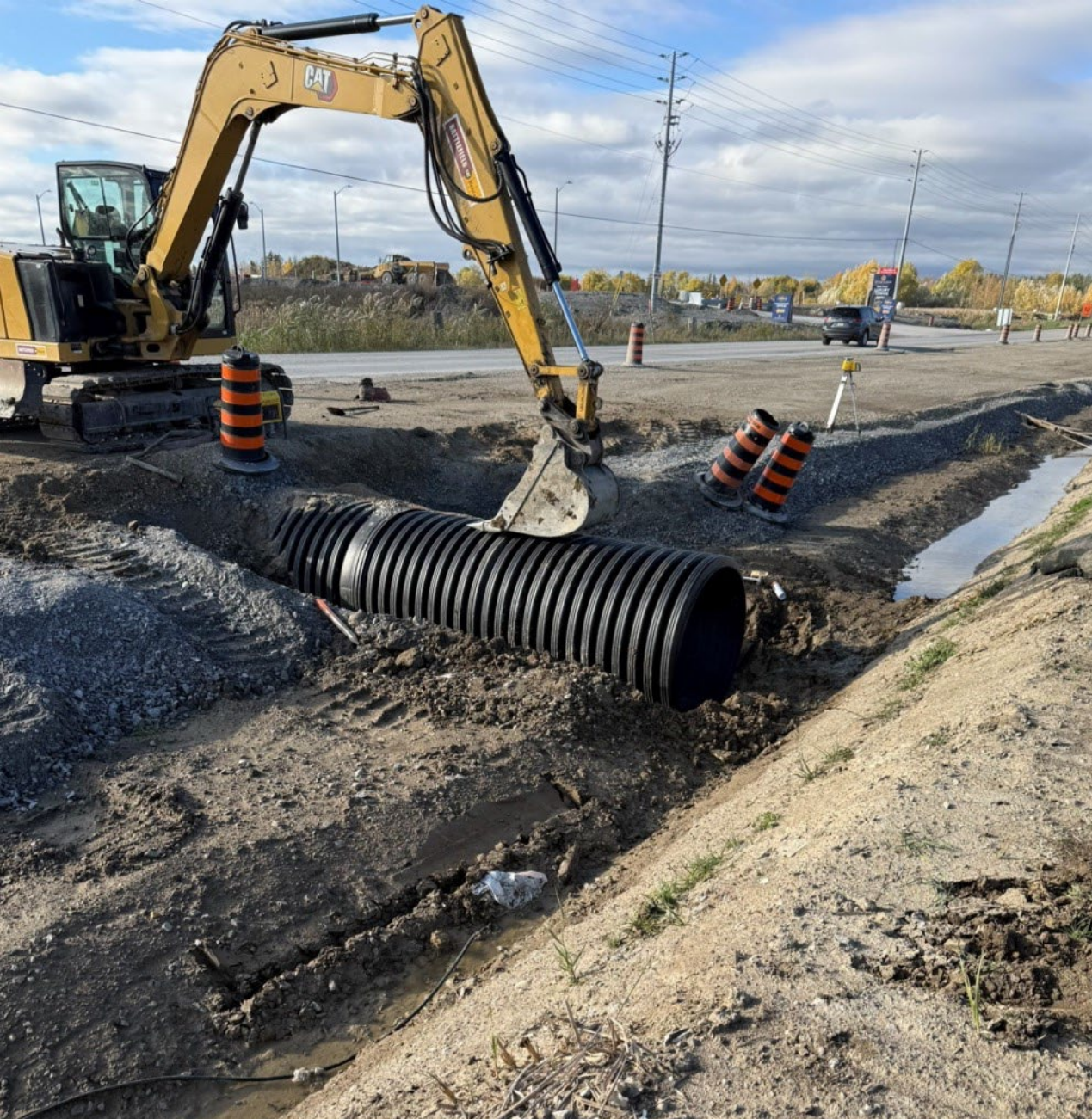
Preparation underway for road widening, including installing culvert extensions and shifting the road, 19 th Avenue, east of Bayview Avenue, City of Richmond Hill
