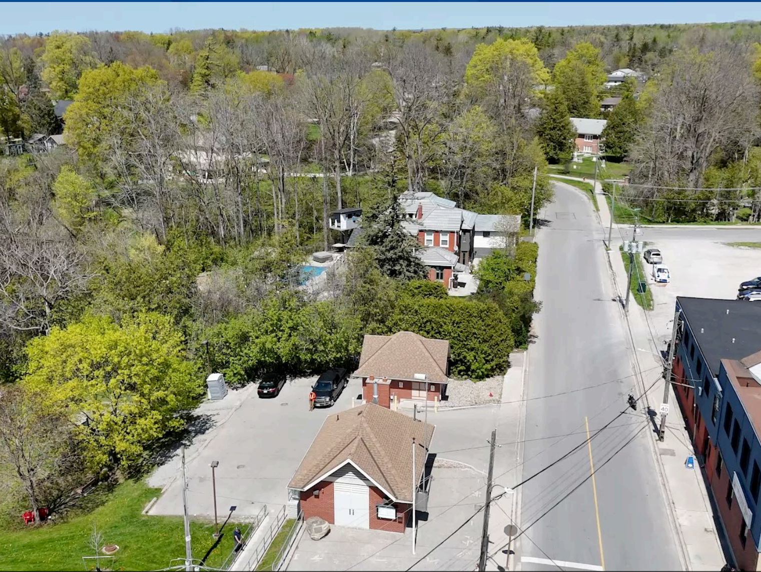
High Street Sewage Pumping Station, Town of Georgia
