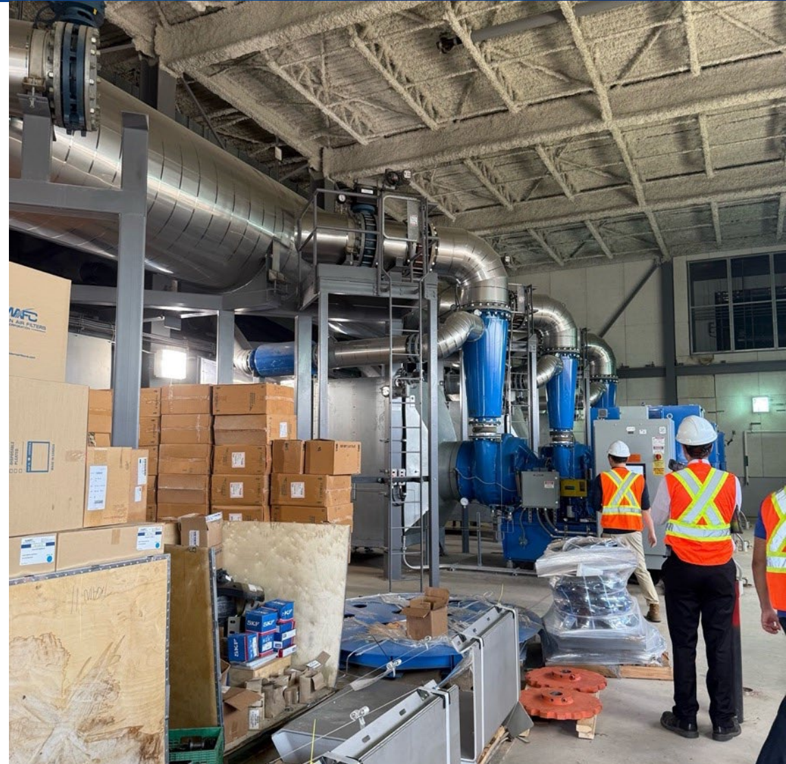
Duffin Creek Incinerators 1 and 2 construction, City of Pickering
