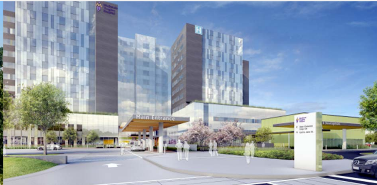
Mackenzie Vaughan Hospital
