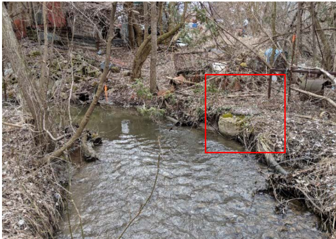
Sanitary Manhole exposed in Patterson Creek
