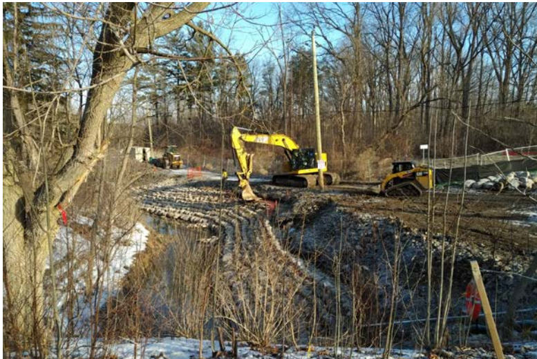
42-metre revetment along Pomona Creek, constructed in 2019
